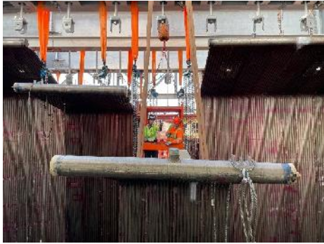
Boiler Panel installation
